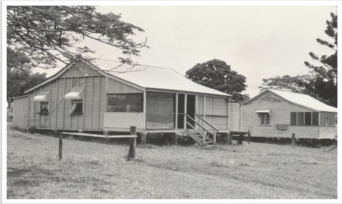
Plate 14.51: These houses at Etowrie on the Northside in 1979 are typical of the many small workers' cottages that once existed around Mackay. The exposed studs on the outer wall were quite usual, and the style was repeated on the verandah inner walls.
