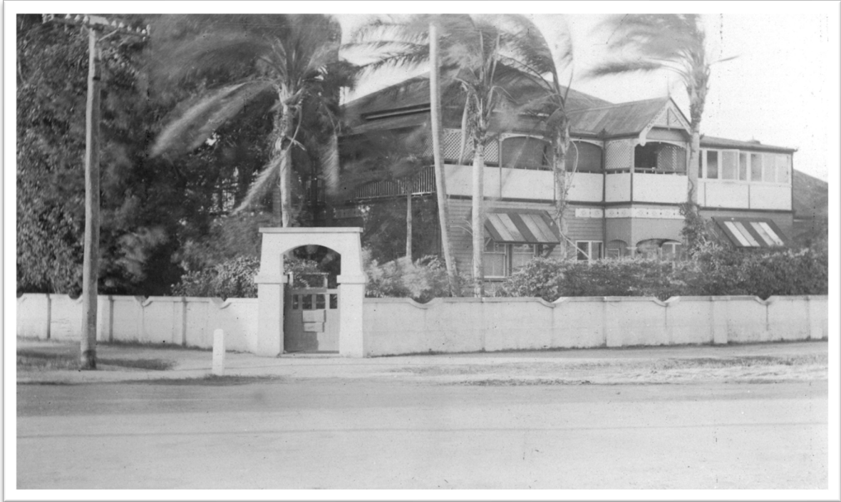
Plate 14.45: Dr C.E. Williams' residence on the corner of Albert (Gordon) and Brisbane streets. Source: State Library of Queensland.
