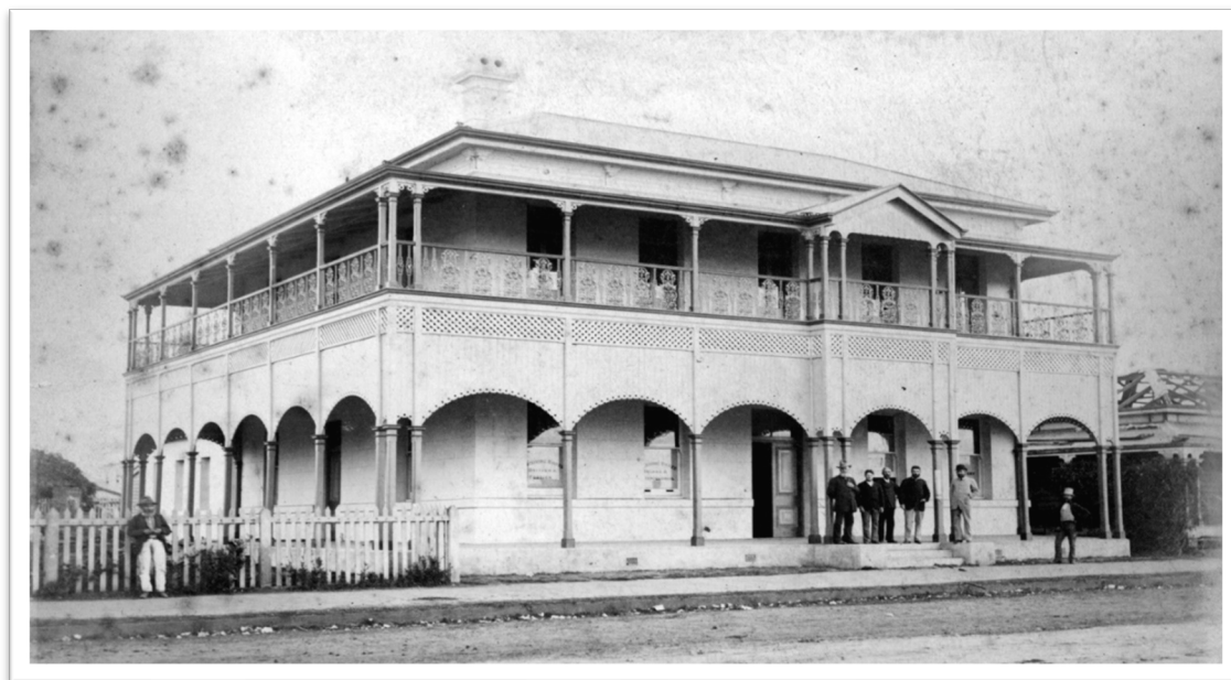
Plate 14.21: The main Post Office was built from masonry in two stages. The building pictured here is the first stage, completed in 1883. It is the left side of the current building (Plate 14.22). The Telegraph Office side and the clock tower were added in 1884. Originally, the lower level was for post and telegraph services, a kitchen, and servants' quarters, while the upper level was the Postmaster's residence. The only other 1880s building of equivalent grandeur was the AJS Bank in Victoria Street, constructed in 1880. Both were designed by the Government Architect Francis D.G. Stanley and were a sign of the growing importance of Mackay.
