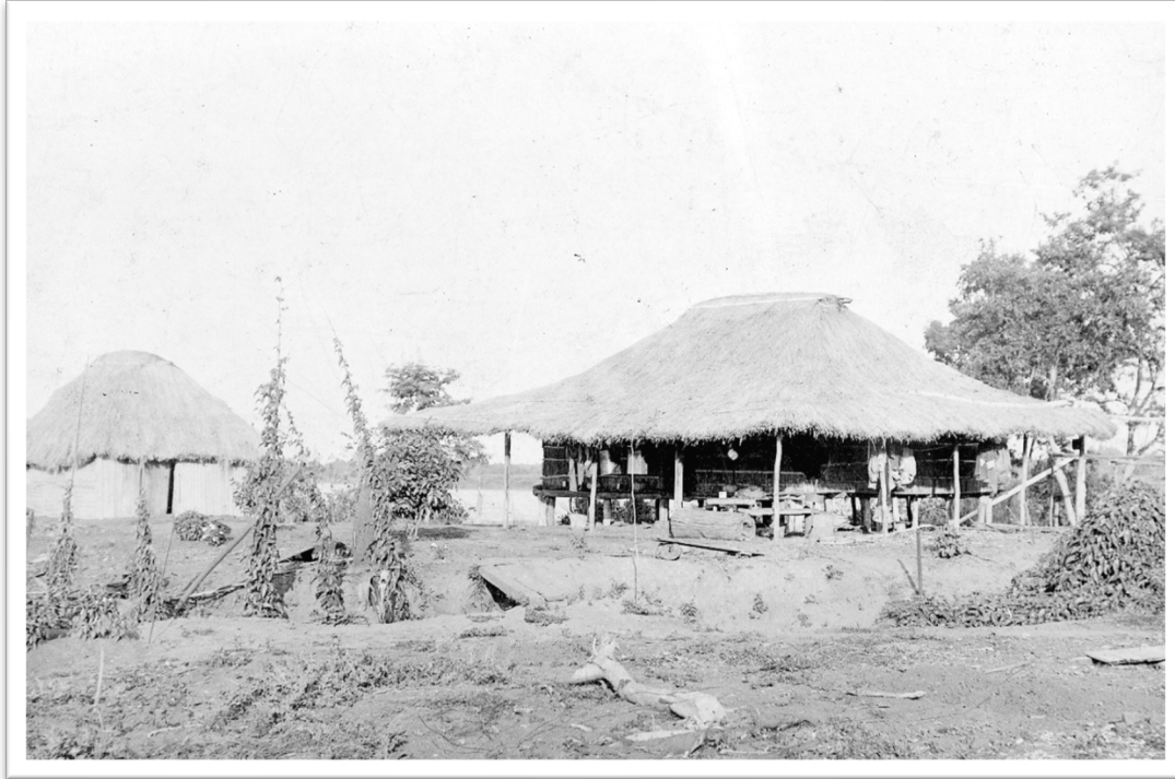
Plate 11.4: A typical Islander house at Mackay, ca. 1890. This home had a spacious overhang, creating a verandah. The thatched roof is made from blady grass, which is also used on the walls, held in place by batons. The smaller building may be the kitchen.
