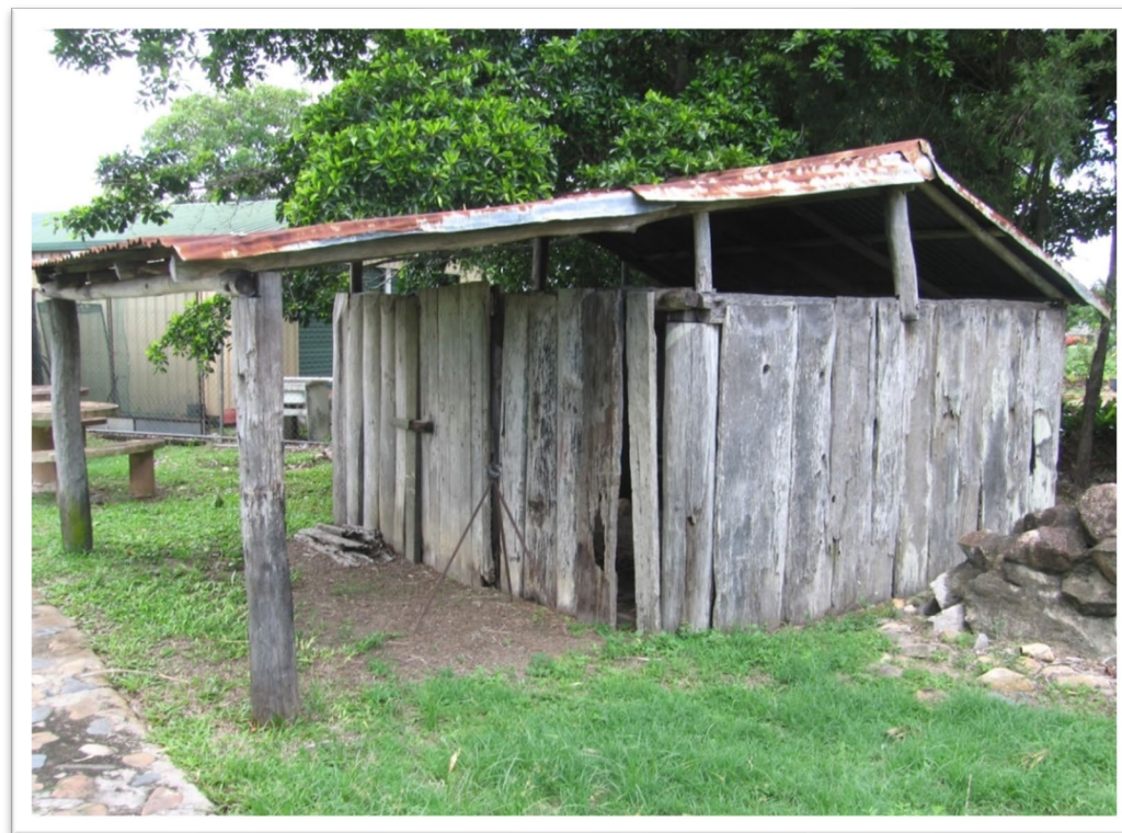
Plate 6.7: The Hamilton structure was moved and is now part of Mirani Museum, labelled as a ‘dairy’. Some of the defence holes are visible in this photograph.
