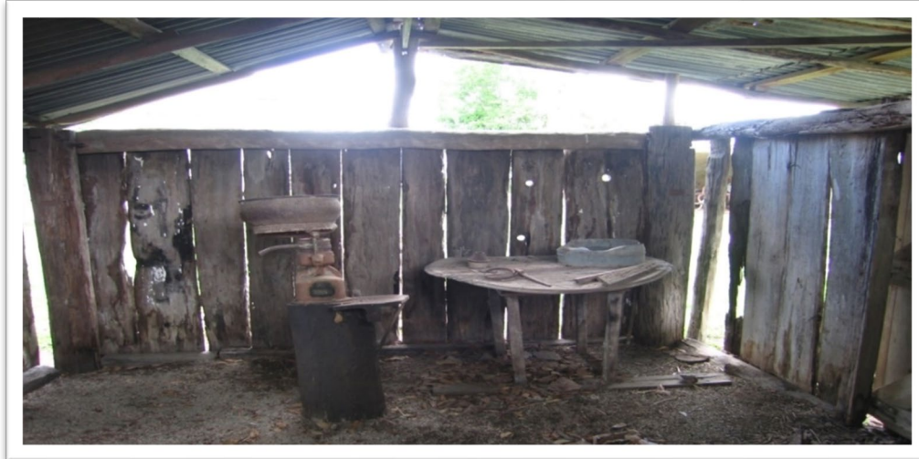
Plate 6.6: Some of the holes in the walls of the Hamilton Station ‘dairy’ are visible in this photograph. The high holes are to look through and the low holes to shoot through. These reoccur around the walls. The boards may once have been part of a larger building, as similar boards with knotholes seem to have been included in what became the slaughterhouse for Hamilton station.
