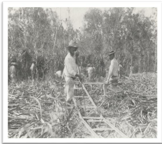
Plate 7.37: Laying portable tramways to transport cut cane from a Homebush field, 1883.
