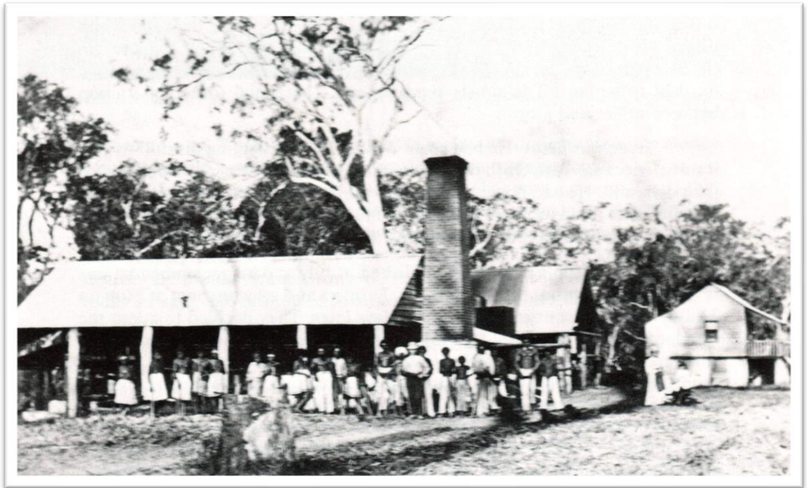
Plate 7.17: Small Cassada plantation mill operated from 1870 until 1886. There are at least eight Islander women in the photograph, which is unusual. Note that the women appear to be only wearing skirts, with no tops. The men are not wearing shirts. This photograph is probably more realistic than the fully clothed Islander photographs from this era.
