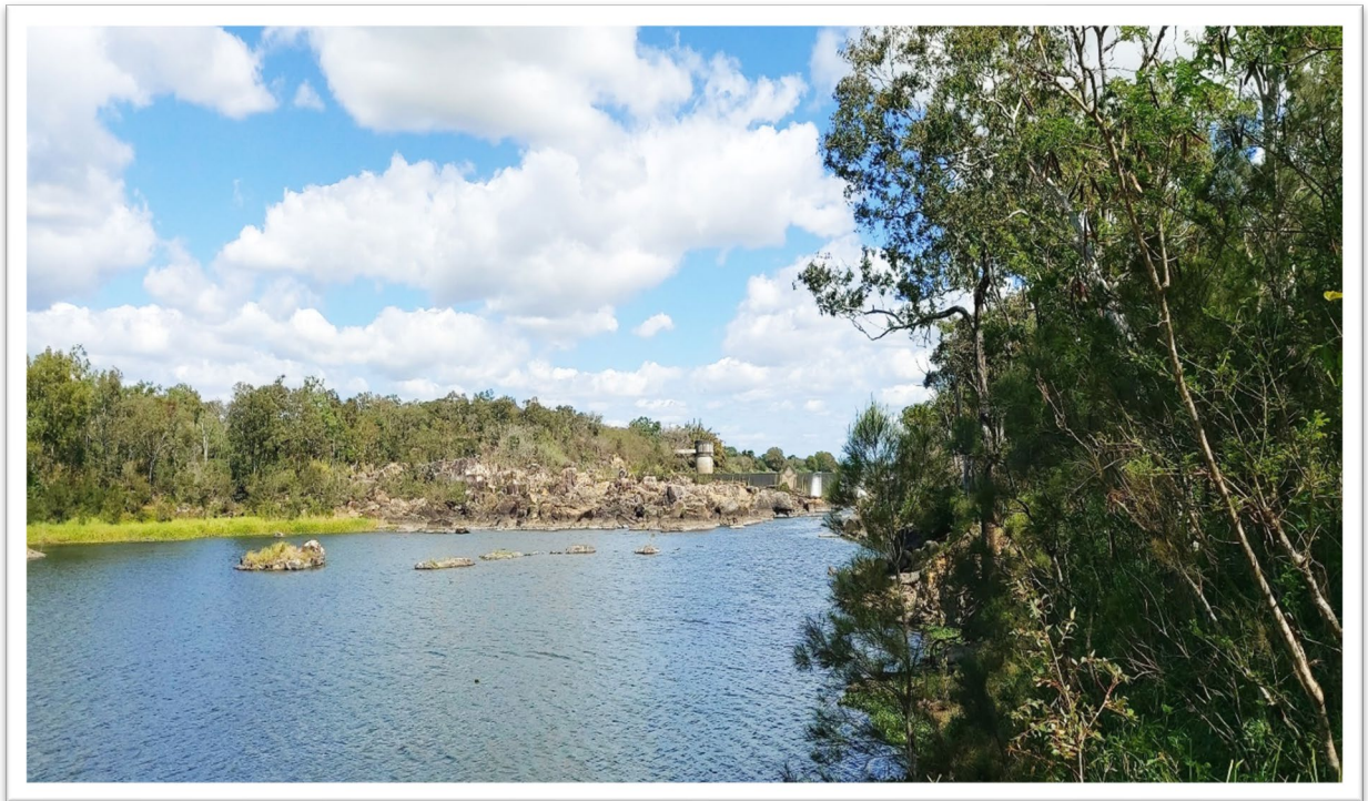
Plate Intro.17: The Pioneer River has several weirs and dams: Marian Weir was built in 1952, followed soon after by Marini Weir. Dumbleton Weir (pictured here) was built in 1982, 15 kilometres upstream, at the point where the saltwater stops, and the fresh water begins. Dumbleton Weir provides water for Mackay. It has been upgraded twice. In 1977, water from the Pioneer River was diverted into Kinchant Dam between Mirani and Eton on the upper reaches of Sandy Creek. Teemburra Dam was constructed in 1997, 50 kilometres west of Mackay at Pinnacle.
