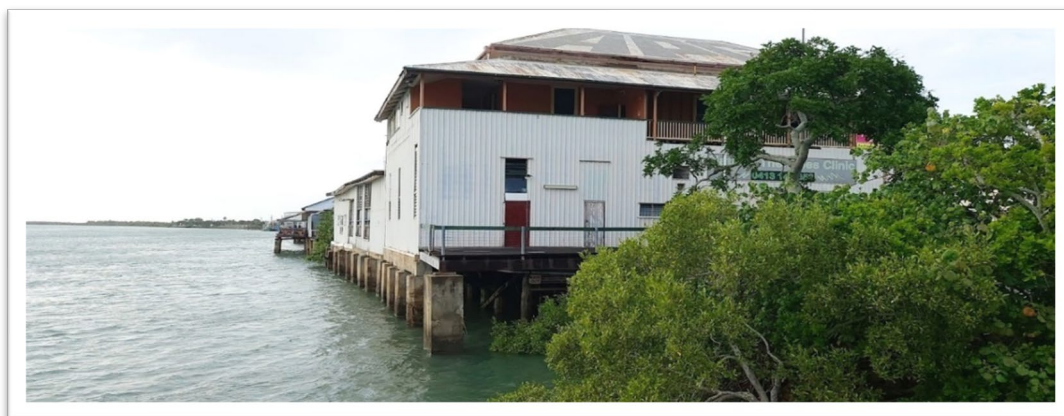
Plate Intro.10: The W.R. Paxton & Co. building on the edge of the river in River Street. The company was founded in 1876 as shipping agents, and a wholesale and retail hardware business.
