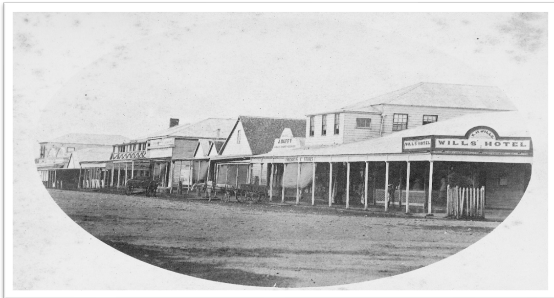
Plate 13.27: Wills Hotel on the northeast corner of Sydney and Victoria streets is in the foreground, previously known as the Royal, the Standard, and Mrs Cooks Royal Hotel. It is on the site of the first building in Mackay, erected by Andrew Henderson in September 1862. Thomas Read owned the hotel in 1864–65, after which it transferred to Jane and James Cook. They sold it to Korah Halcomb Wills in 1870, who used his surname as the hotel's name. Jane Cook moved a few doors down Sydney Street towards the river and built another Royal Hotel; its upper crossed railings can be seen in this photograph. Wills sold out in 1882, although his name remained on the hotel. P. Michaelis's store is next door, then J. Duffy's bakery and grocery. The photograph is from the 1870s.
