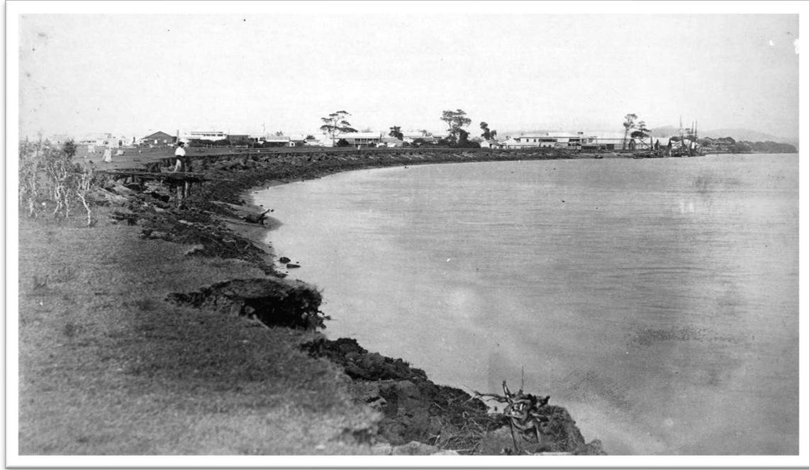
Plate 13.8: The banks of the Pioneer River were constantly eroding and difficult to use as a major port. This 1870s photograph, taken from the coastal end, shows the early wharves. The river is tidal and was always too shallow to berth large vessels.
