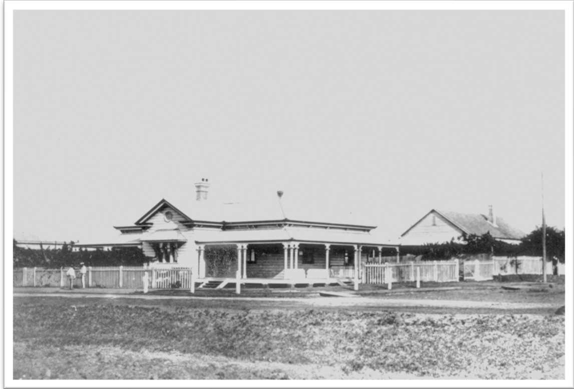
Plate 13.32: The Mackay Post Office and residence were designed by the Government Architect Francis D.G. Stanley in 1874, although construction was delayed, and the buildings did not open until 1877. The buildings were on the same site as the new Post Office which was built in 1883–84 (Plate 14.20–22). The original buildings were moved next door to be used as the Customs House.
