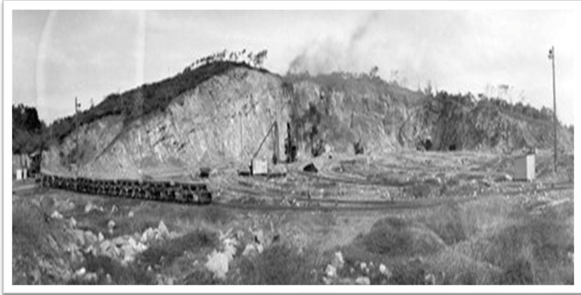
Plate 13.14: The mining of granite from Mt Bassett quarry, used to create the outer harbour. Source: State Library of Queensland.
