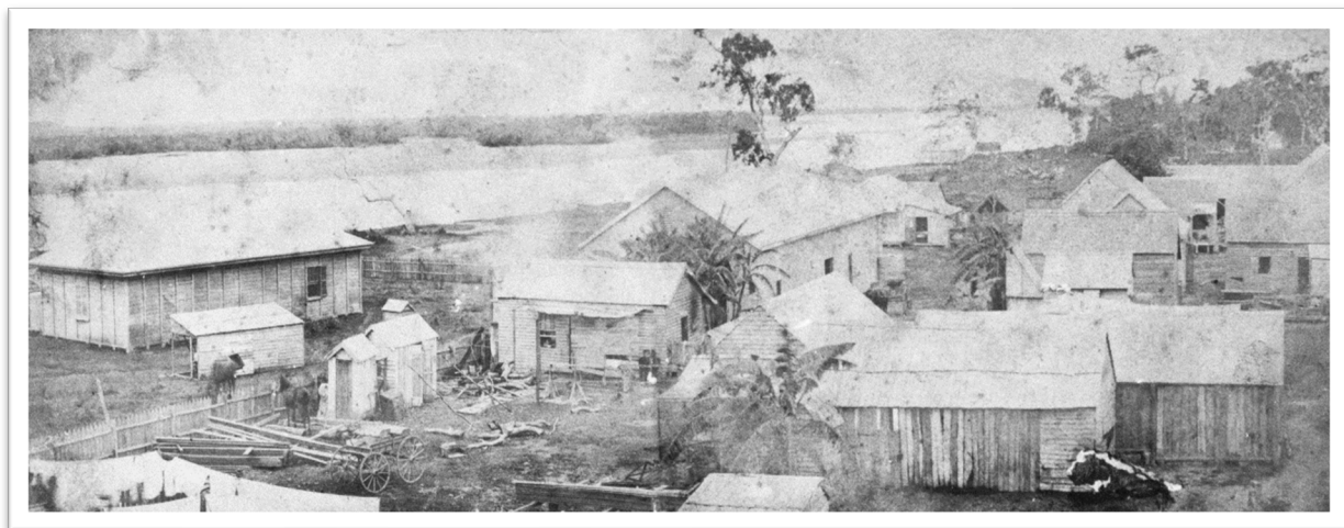
Plate 13.3: Another view of Mackay in 1868. The Court House is on the left on the bank of the Pioneer River, and a butcher shop, general store and stables are towards the right at the river end of Sydney Street. Several outhouses can be seen, and washing is hanging on a line in the bottom left.
