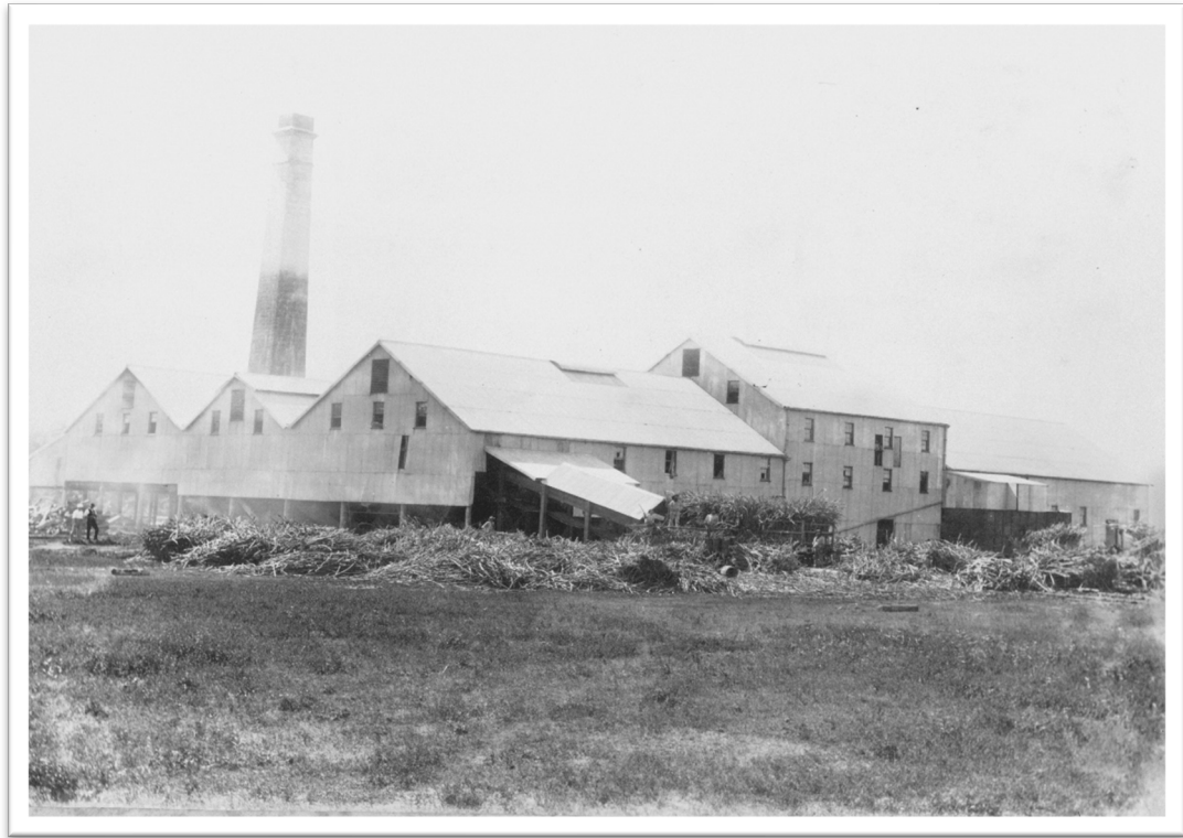
Plate 10.12: Racecourse central mill first crushed in 1889.
