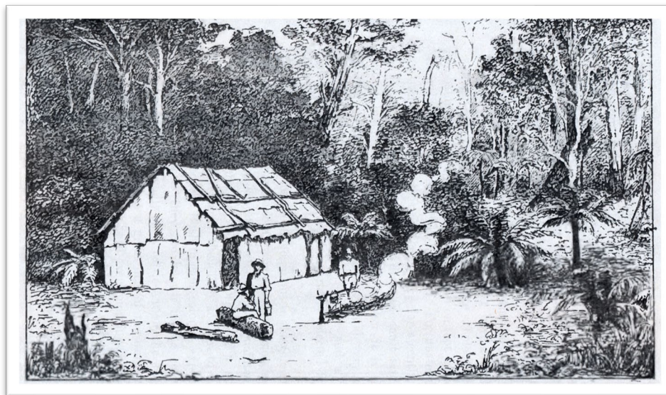
Plate 4.35: Out-stations were always primitive, consisting of a hut and a series of stock yards, aimed to make cattle management easier, but usually not for permanent habitation. This out-station was on a pastoral property, presumably on the Blue Mountain or Mt Spencer runs in the 1880s. The house is made from saplings and bark sheets, tied together with hide strips. The cooking was done out in the open. Source: Finch-Hatton 1886, 77.
