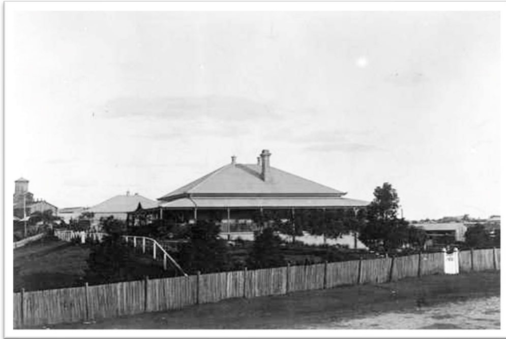
Plate 4.27: ‘The Hollow’, Charles and Wini Rawson’s house on the river at the Teneriffe end of Merthyr Road, New Farm, Brisbane.
